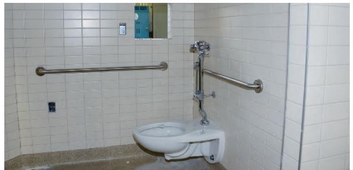
*The finished bathroom pods arrive at the job site with toilet, sink and other fixtures in place and ready to use once the final piping connections are made.*
